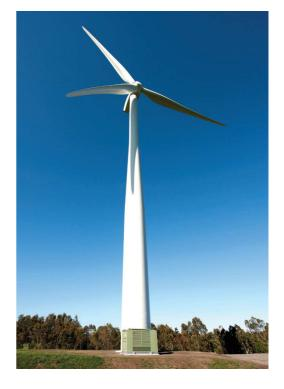
WTG Transformer kiosks complete with internal MV switching and full 690V LV frames. In less than six months the units were designed, tested, type tested and shipped to site, on time and in full.
